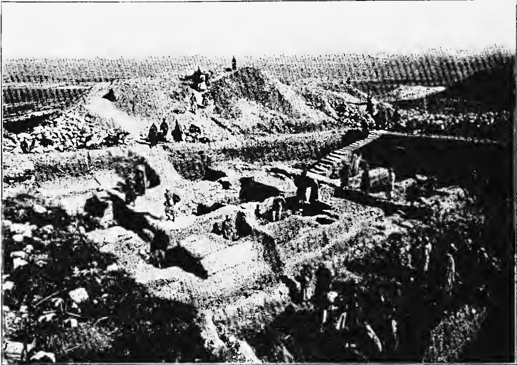
FIG. 58.—LARGE BRICK BUILDING IN IIIa
